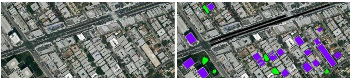
Figure 6: Scene with high density commercial areas and a large road in the middle.
